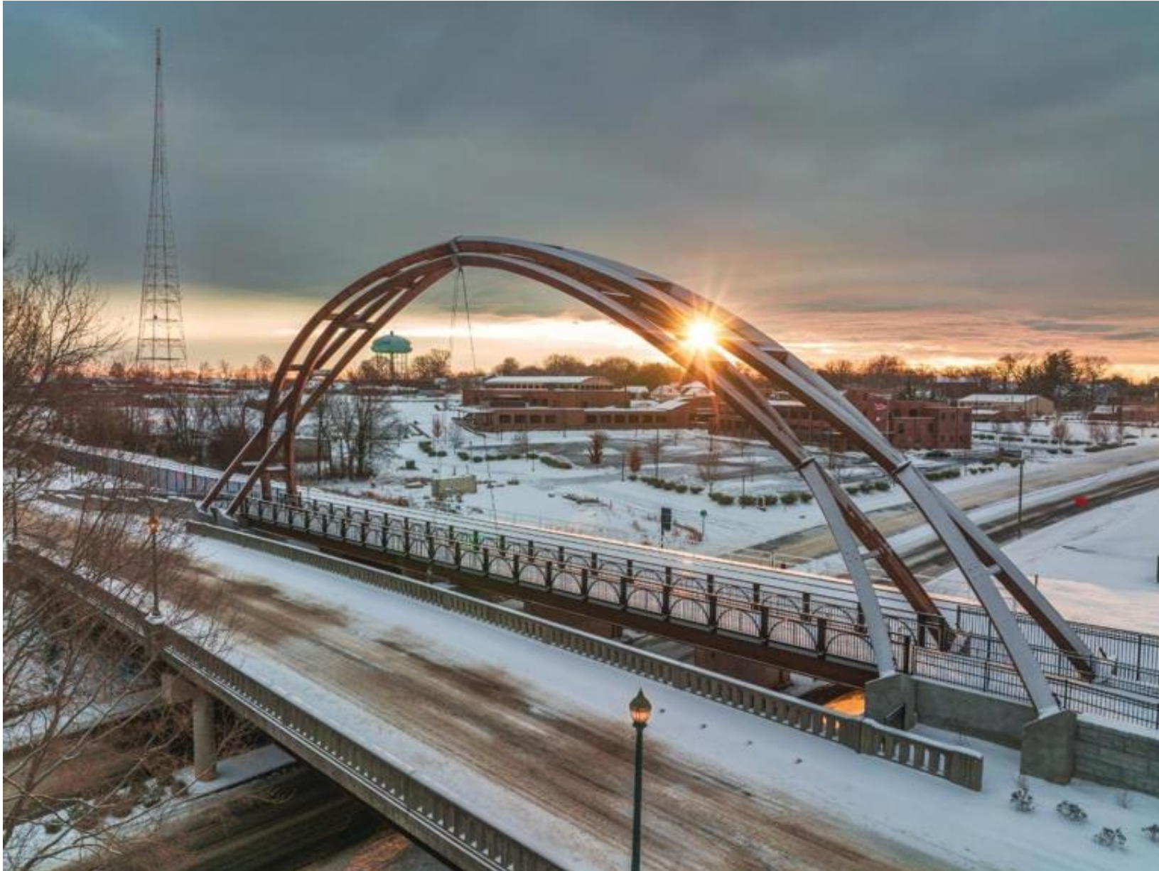
Photo obtained from https://www.thestructuralengineer.info/news/north-carolina-a-pedestrian-bridge-collapses-video-reveals-the-arches-collapsing Source: Nelson Aerial Productions
